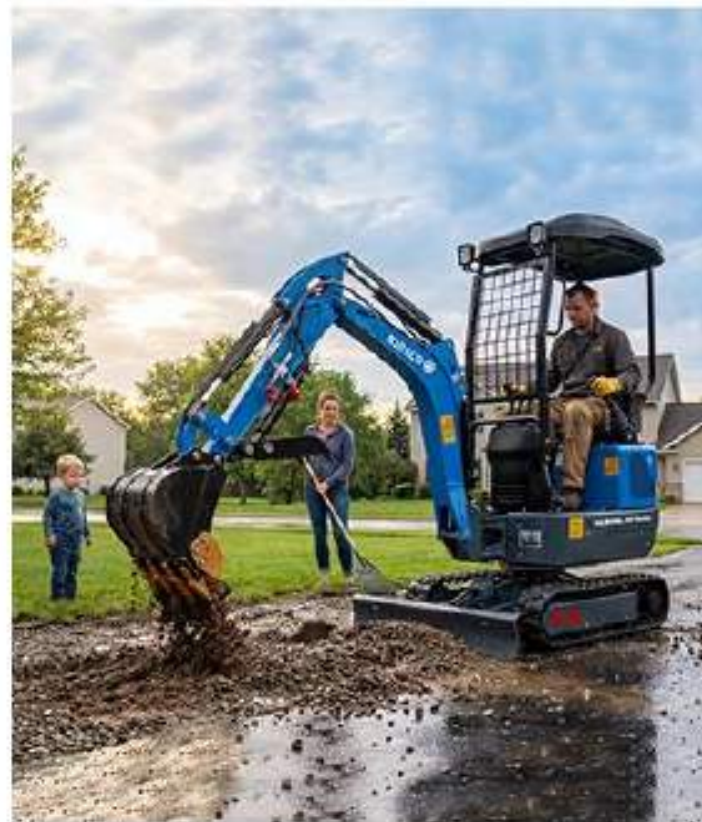
REPAIR A DRIVEWAY
