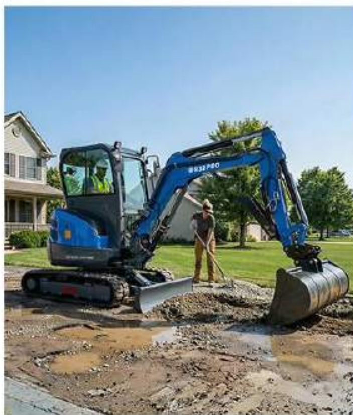
REPAIR A DRIVEWAY
