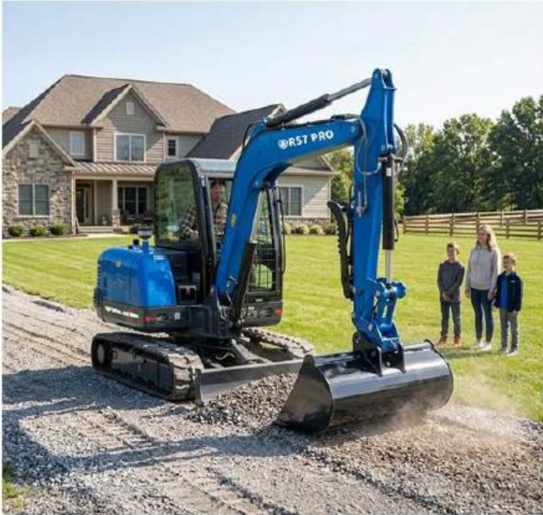
REPAIR A DRIVEWAY
